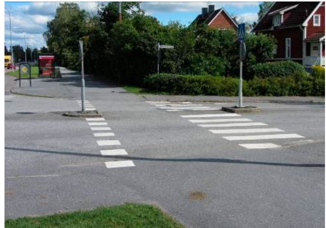
Junction before being rebuilt
