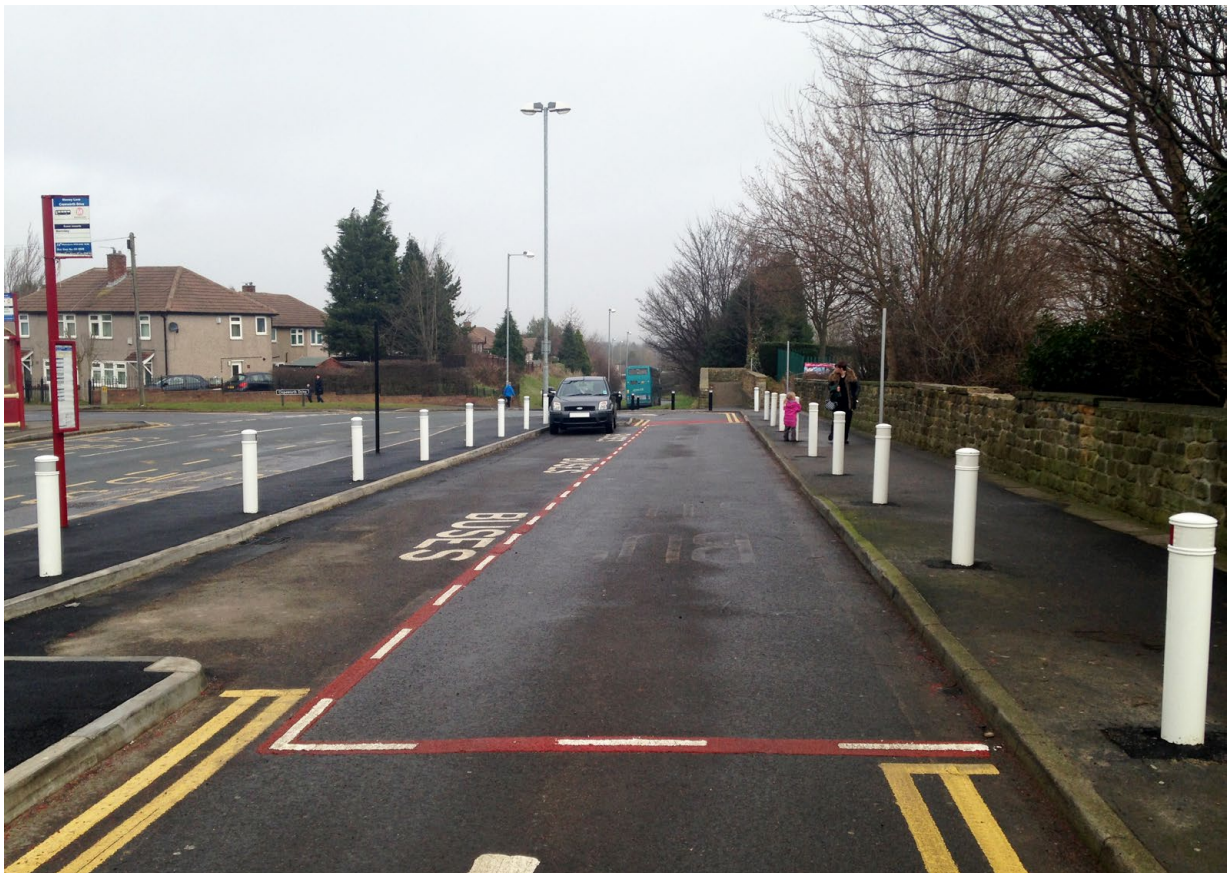
Improved bus layover facilities in Wakefield, funded under the “Bus Hotspots” programme Photo: WYCA
